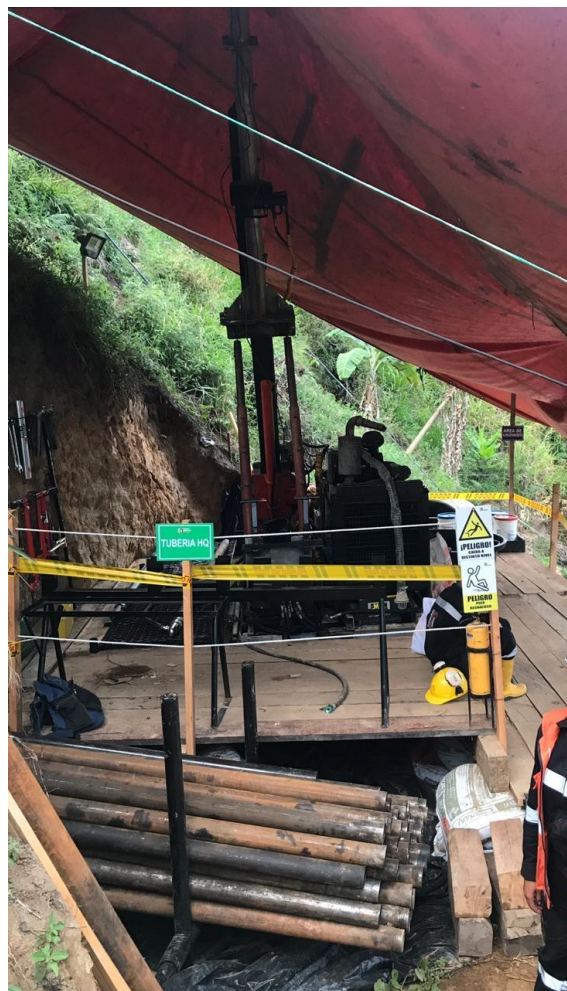
Drill Platform and rig at Chuscal 30/09/2019
